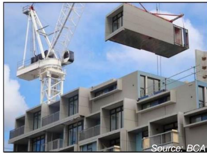
PPVC module installation
