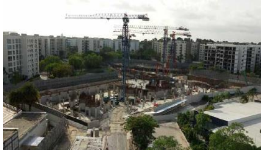
Construction projects at The Jovell and Martin Modern
