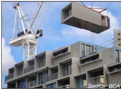
PPVC module installation
